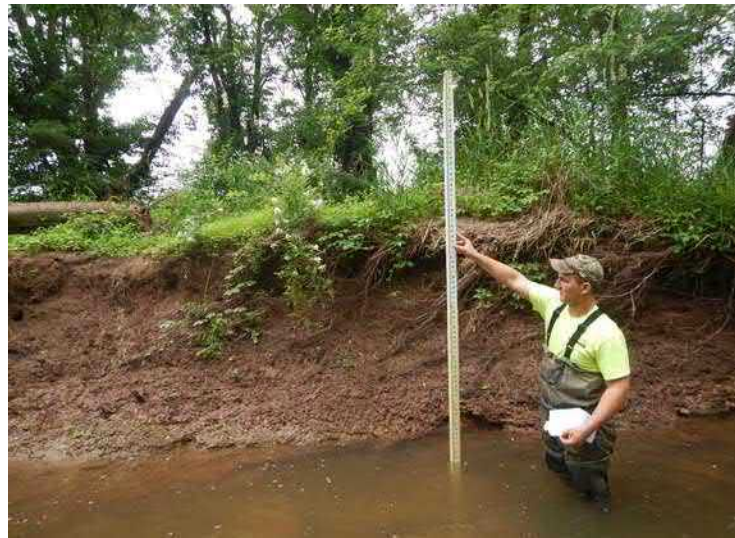
Existing Conditions Photo
