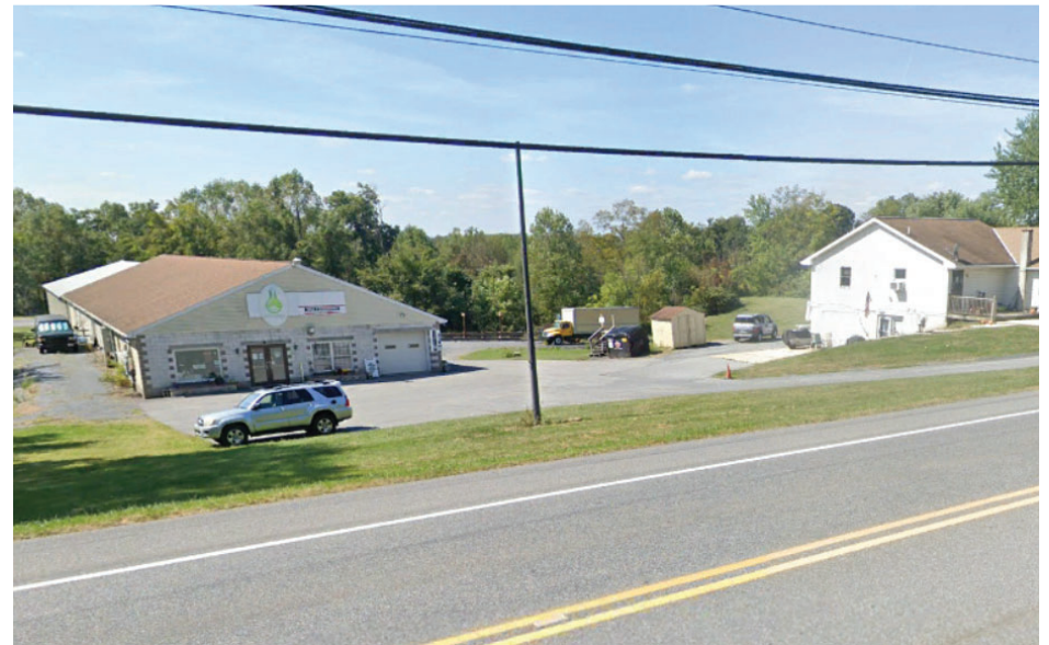
The image above depicts existing low-density commercial development along Route 230. Future land use goals should include targeting areas for continued commercial, industrial, and mixed use development in the central section along State Route 230 and 283.
